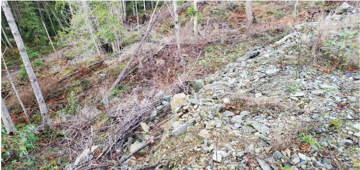
Photograph – Existing end-dumped Fill Slope above Priestland Road (Sta. 0+380 to 0+500)
