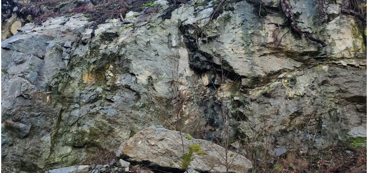
Photograph – Bedrock Cut above Priestland Road (Sta. 0+260 to 0+340)
